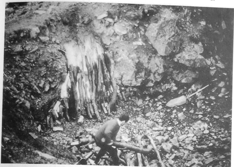
FIGURE 2.5 Firesetting experiment in progress at Cwmystwyth, central Wales. A fire of substantial logs was left to burn for many hours against the face to be mined.
