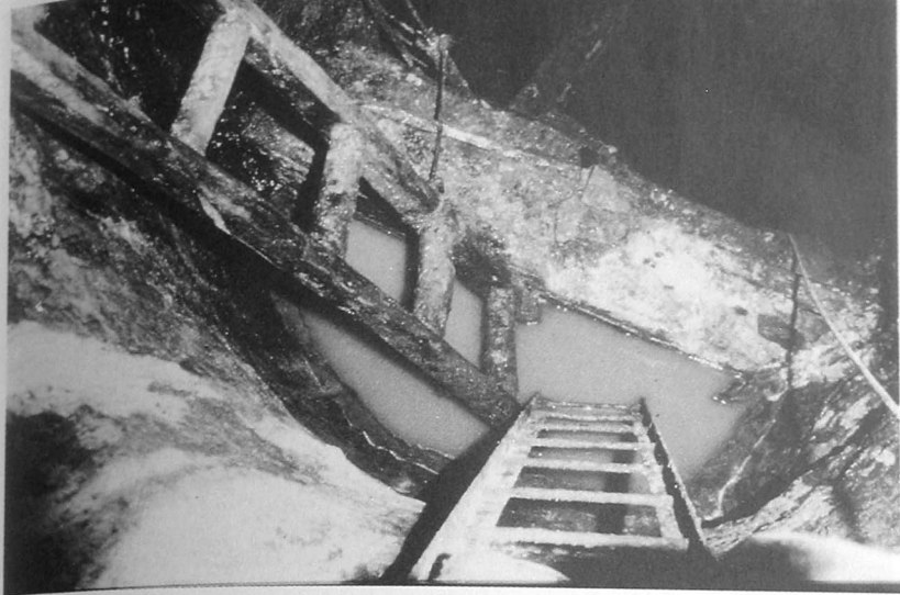
FIGURE 2.39 Wooden bailing dam in the side of a shaft at Dariba, dated to the third century BC. The ladder on the right is modern, that on the left is ancient.
