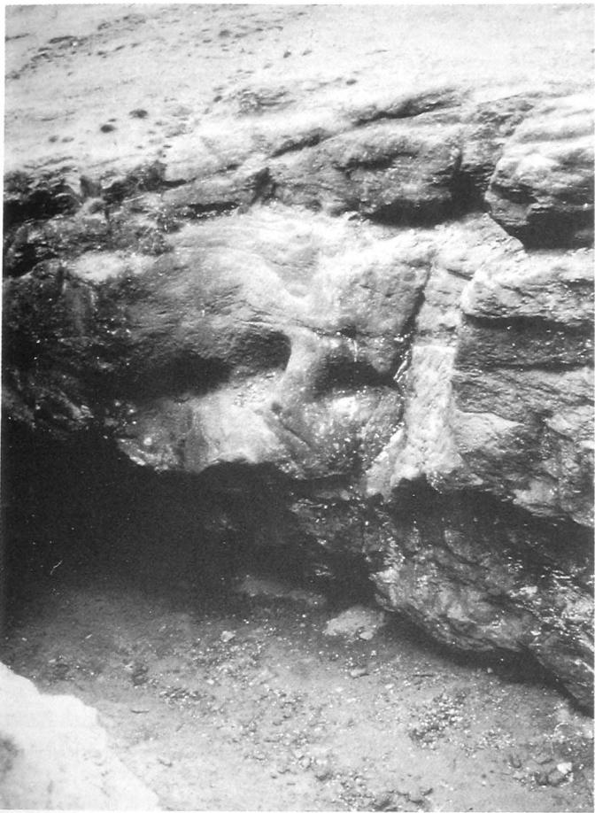
FIGURE 1.1 Four thousand years of mining history in one rock face, Engine House Lode, Alderley Edge, Cheshire. The diffuse pecking in the centre made by stone hammers in the Bronze Age, a small shaft to the right cut with steel stools, probably post medieval, and the jagged edges of the main trench caused by blasting in the nineteenth century.
