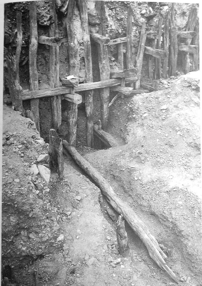
FIGURE 2.48 Section of major timber revetment running along one side of the opencast shown in Figure 2.46. The horizontal beam exposed in the foreground held a similar revetment on the next bench down. (The white rectangle is 10cm long.)
