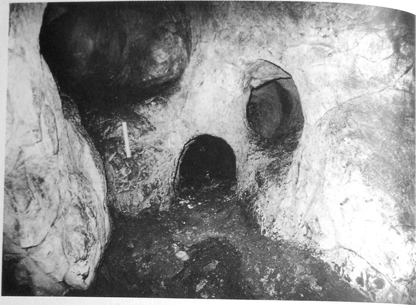
FIGURE 2.6 Complex fireset working at the Kestel tin mine dating from the third millennium BC. Note the smooth continuous contours of the walls, and the very precise nature of the work quite typical of firesetting.
