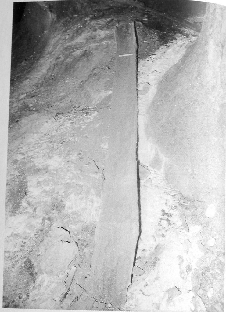
FIGURE 2.38 Drainage channel at Zawar made from a hollowed tree trunk and used to channel water to points where it could be collected and carried out of the mine.
