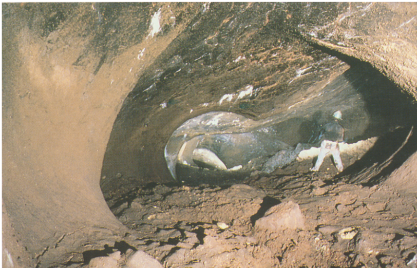
Figure 3 Driving a working forward by successive firesets can produce a very distinctive sinuous profile. Galleries in Zawar Mine.
